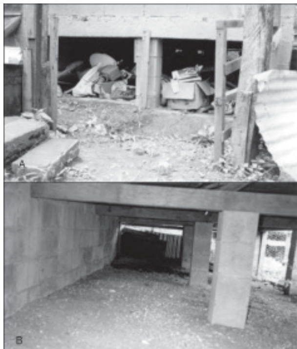
Fig. 2: space beneath house 12. A: before intervention; B: after intervention.
